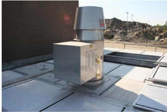
Figure 4. HAWKESBURY BIOFILTER ODOUR CONTROL UNIT.
