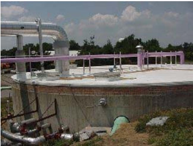
**ATAD Reactor with Foam Control (Lower Left of Picture)**
