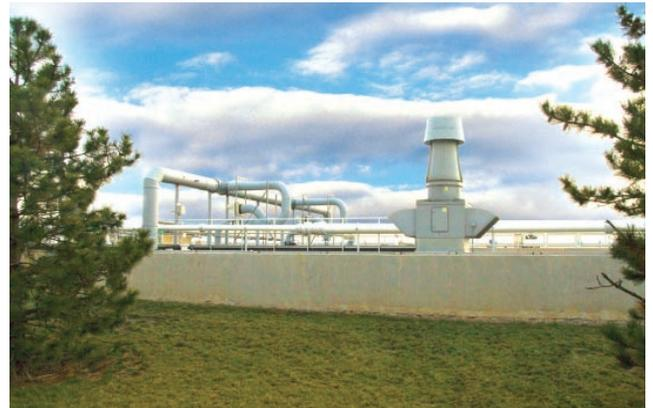
*The Bowling Green, Ohio BiofiltAer biologically removes odors from several potentially odorous sources, including ATAD operations, thermal drying, dewatering building, and the solids storage building.*
