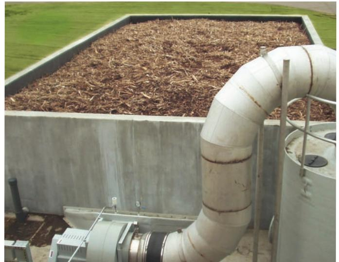
*Marshall uses a rectangular, open top BiofiltAer<sup>™</sup> PLC controls adjust the fan speed to keep the BiofiltAer at an optimum temperature and humidity for biological activity.*
