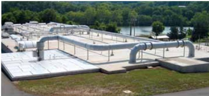
*2010 plant upgrades included the reuse of inactive activated sludge aeration basins. They now house the ThermAer process.*
