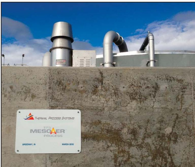
*"We've always credited the conditioning that the biosolids receive in the MesoAer-T as the reason we have excellent decanting ability in our long term storage tanks. This has allowed us to thicken our biosolids without the cost of chemicals and has cut our land application hauling almost in half."*
