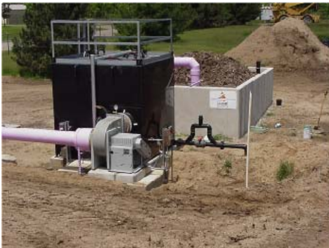
Figure 3 Biofilter With Humidification Chamber
