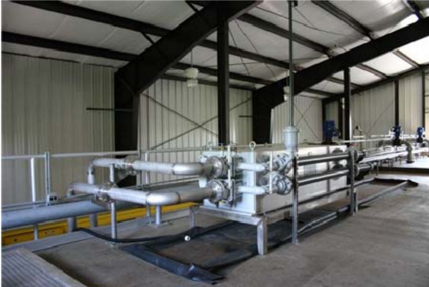
Figure 7 Yorkville IL Cold Water/Biosolids SNDR Heat Exchanger
