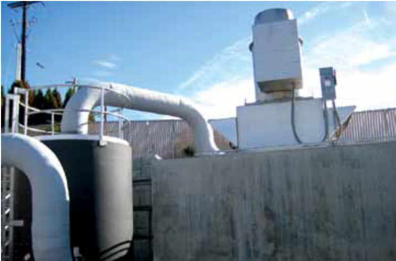
Odors are a big concern for this facility. A BiofiltAer ensures no offensive odors are on-site.
