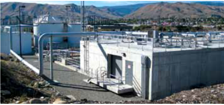
Due to limited space on-site, existing infrastructure was employed to accommodate the new reactors.
